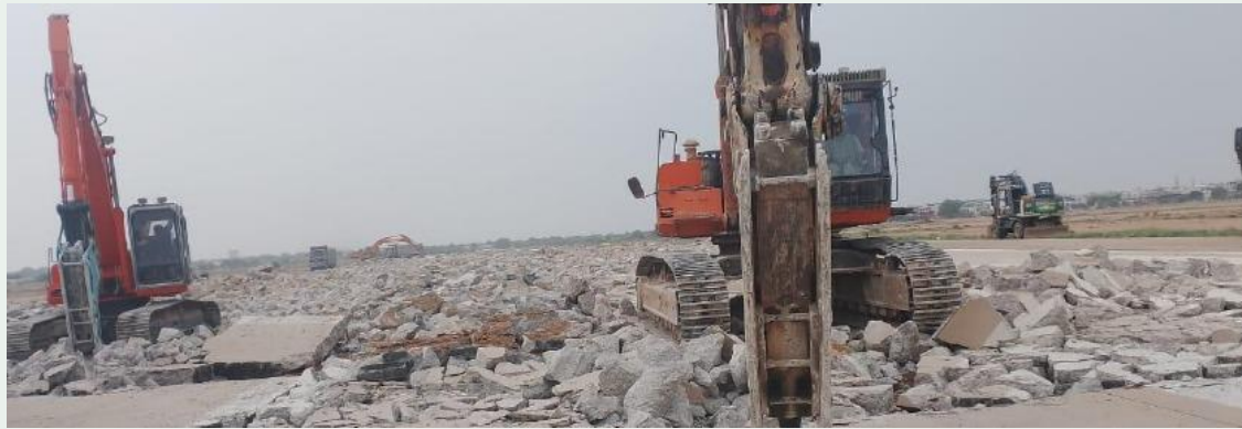
Pavement dismantling & reconstruction interface
