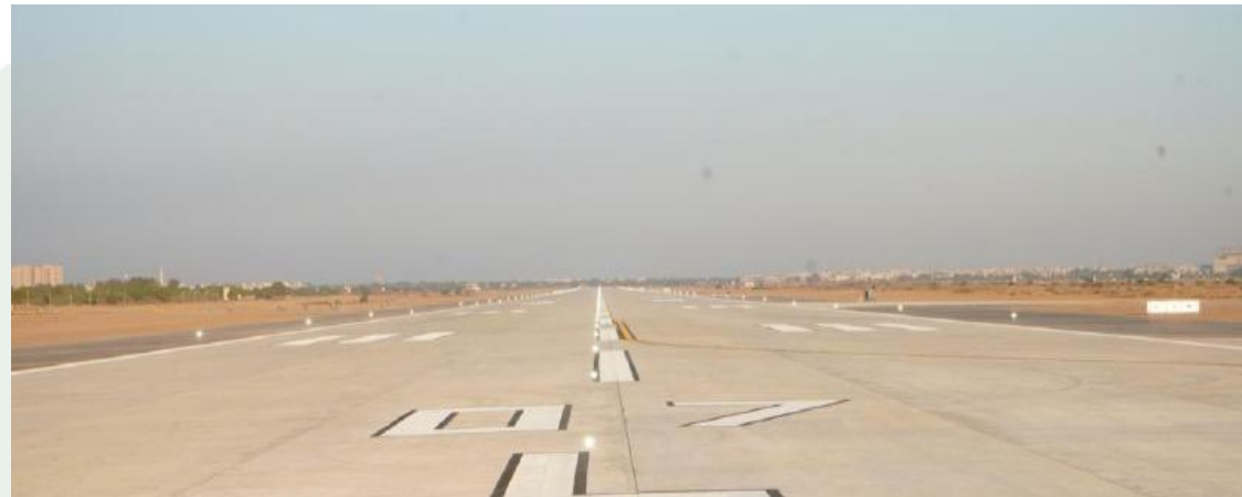
Reconstructed runway surface
