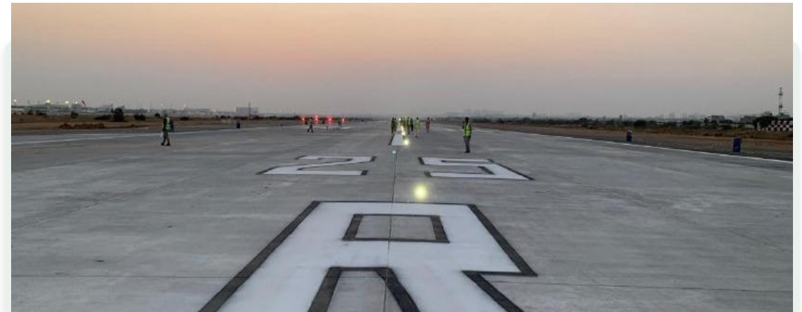
Final surface — markings & lighting (25R)
