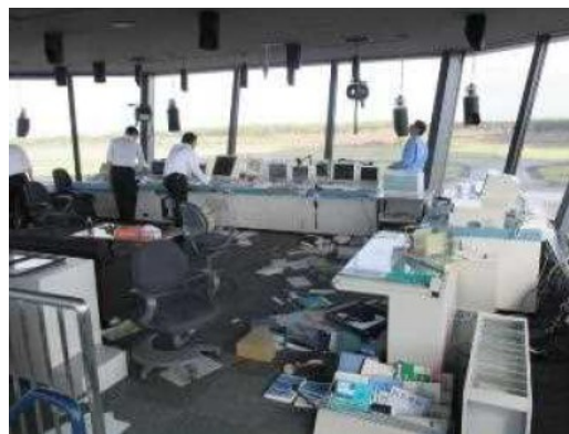
Damaged Control Tower
