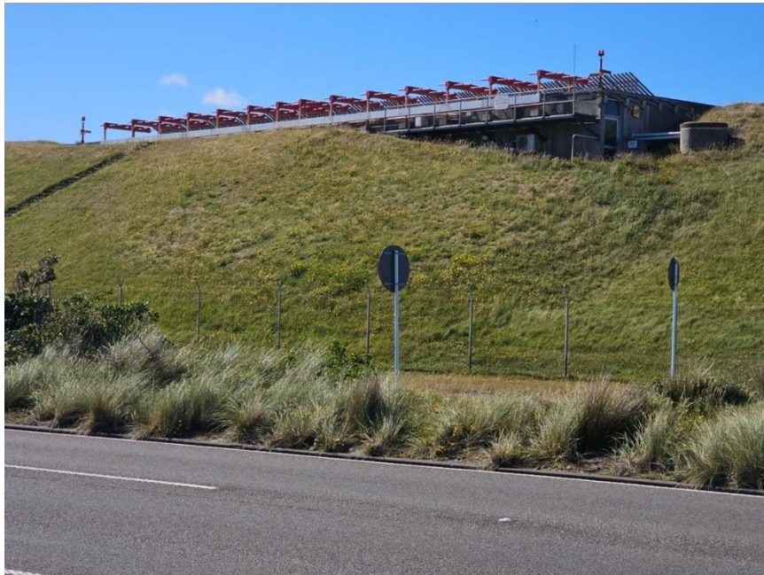
WLZ – LLZ (Localizer) bunker
