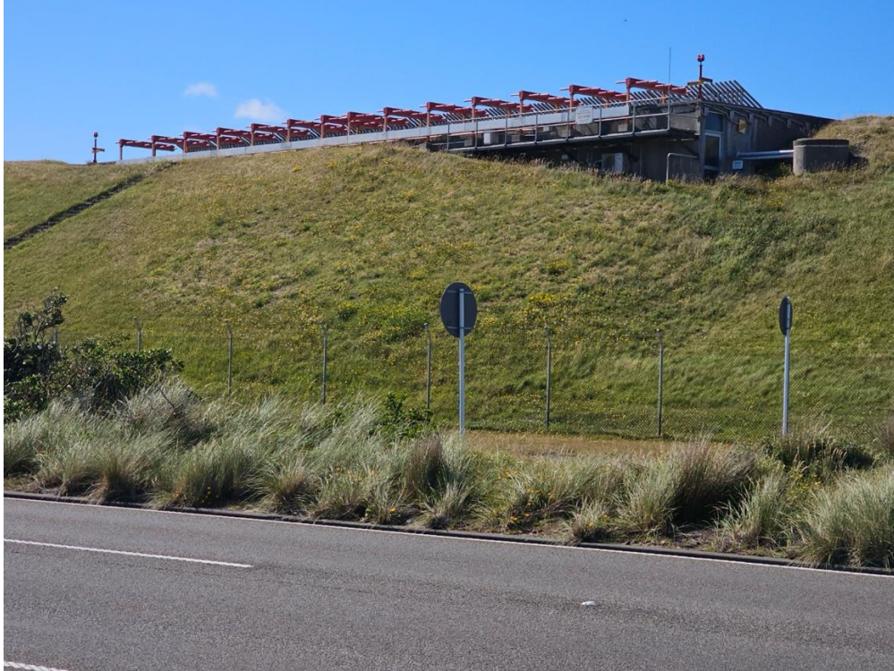
WLZ – LLZ (Localizer) bunker
