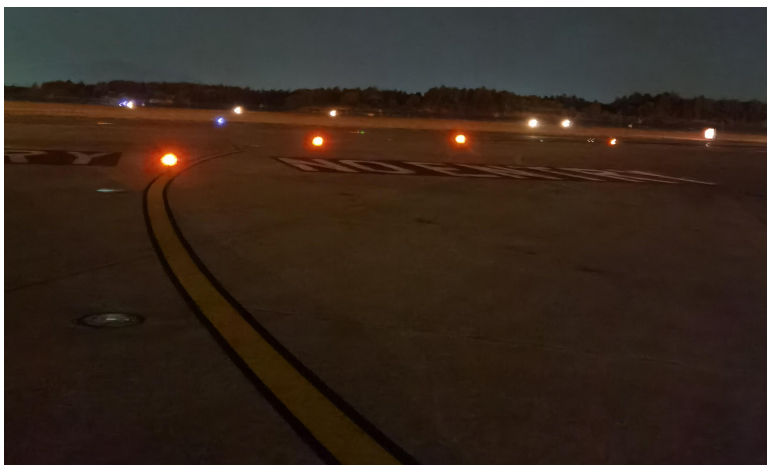
Comparison before and after the A4 taxiway renovation at Changbei Airport
