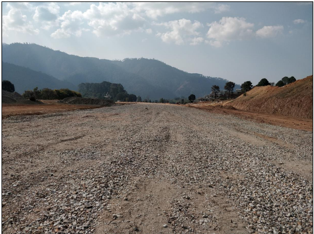
Figure 5.1 – Uncompacted gravel runway with loose stones
