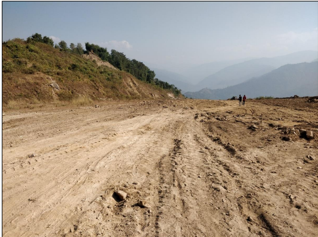
Figure 4.3 – Unserviceable runway due to hardened tyre imprints
