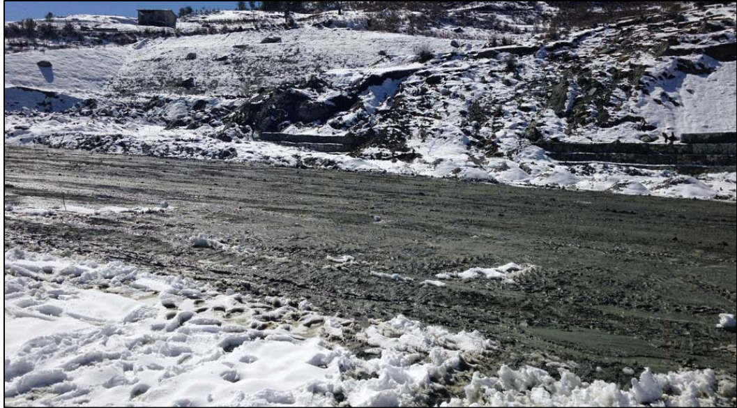
Figure 4.3 – Unserviceable runway due to melting snow
