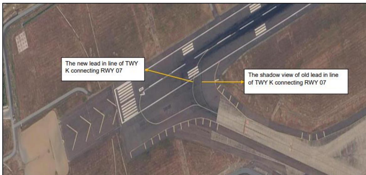
Figure 2. Previous and revised Taxiway K lead-in marking connecting to Runway 07.
