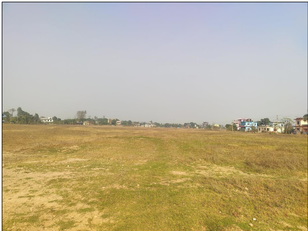
Figure 4.2 – Uneven runway surface
