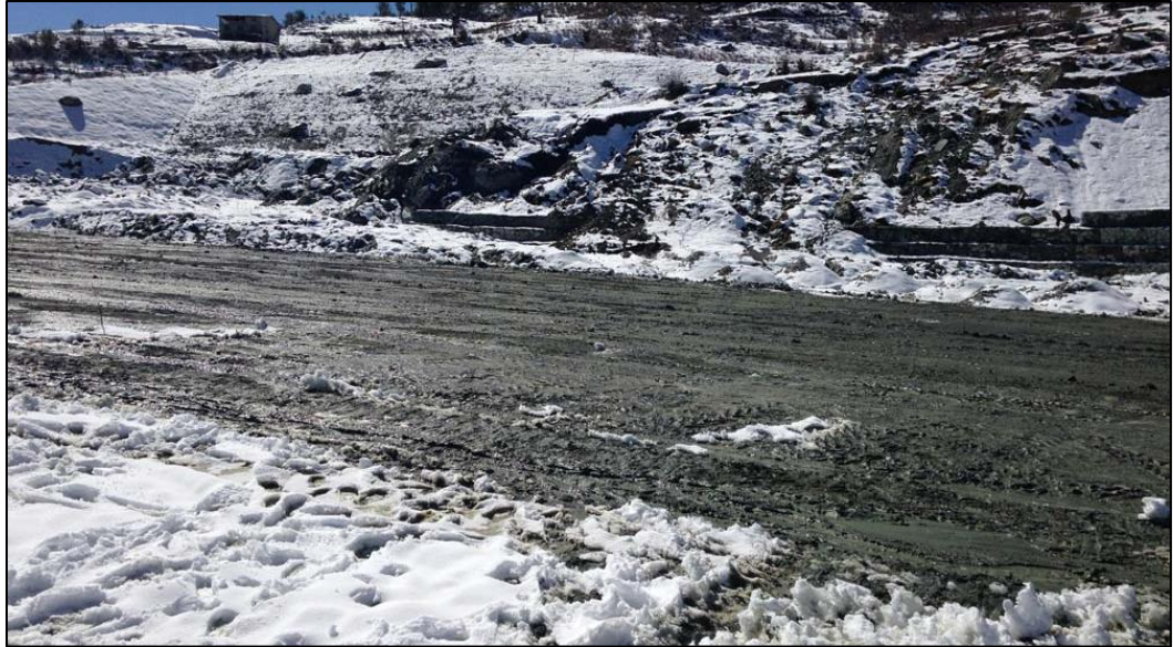
Figure 4.3 – Unserviceable runway due to melting snow
