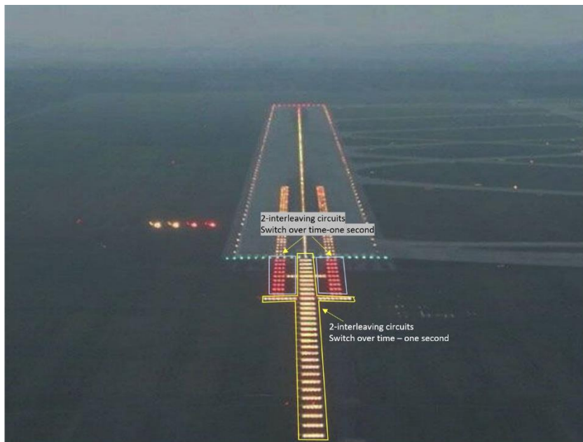
Fig 7. Option 1: Provision of one second switch over time for entire approach lighting system
