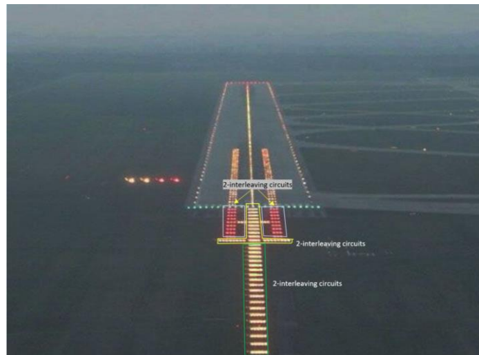
Fig 9. Required circuit design with inner 300 m switch-over time one second, side row barrette lighting (2 circuits) & inner main approach lighting system (2 circuits) and approach lighting system after 300 m (2 circuits) as per present standards referring to Table 8-1.
