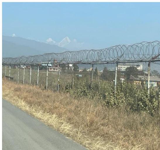
Figure 3: Non- Frangible security fence
