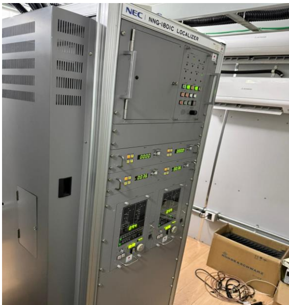
Figure 5: ILS Hut with equipment
