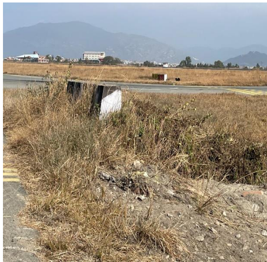
Figure 2: Elevated side wall near taxiway strip
