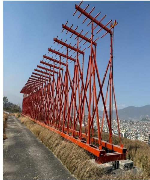
Figure 4: ILS / Glide path antenna and equipment on the runway strip
