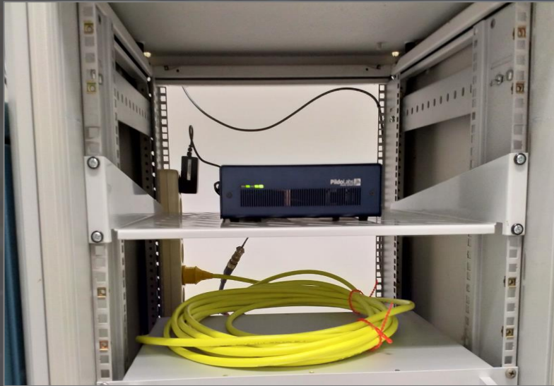
Example of installation of ADS-B Box in a technical rack
