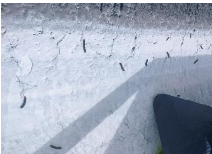
Plate 03:- Caterpillar on runway
