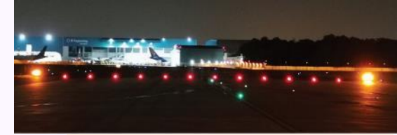
24/7 Stopbar Lights at all Runway entry and exit taxiways & Runway Guard Lights
