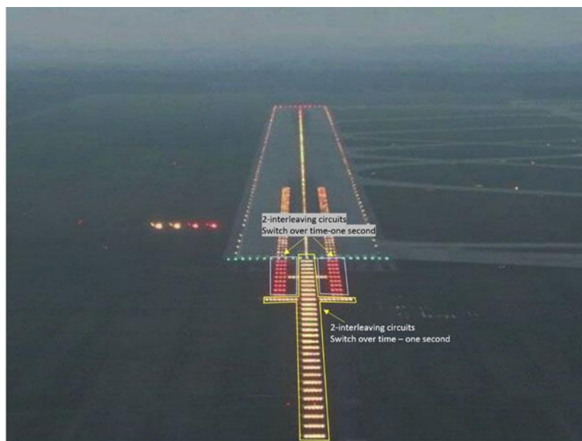
Figure 2: Provision of one second switch over time for entire approach lighting system (Option 1)
