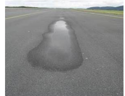
Rutting (High Severity)
