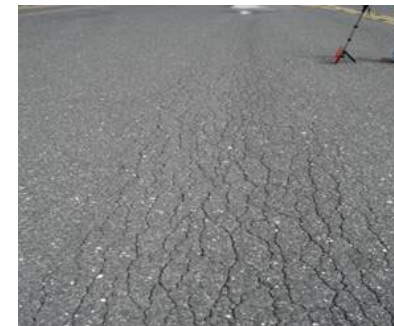
Alligator Cracking (Medium Severity)
