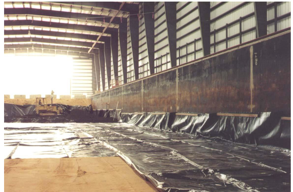
20 mil membrane on the floor of the low-strength subgrade
