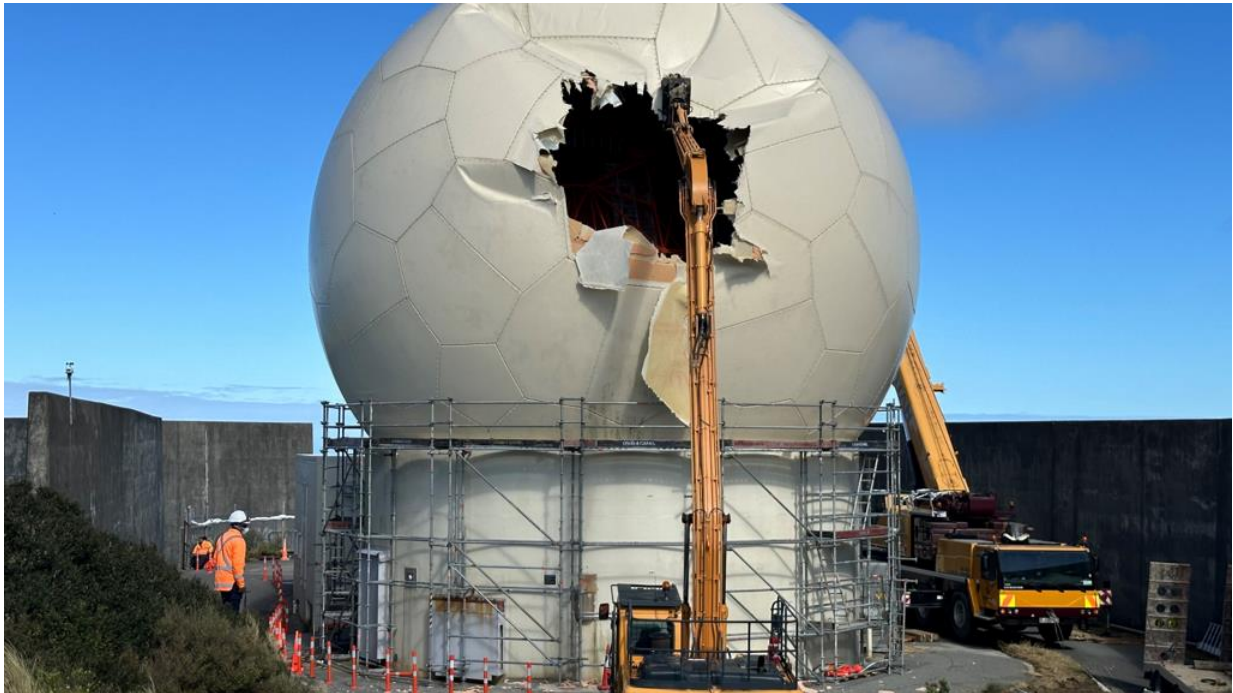
Removing radome using a demolition cutter
