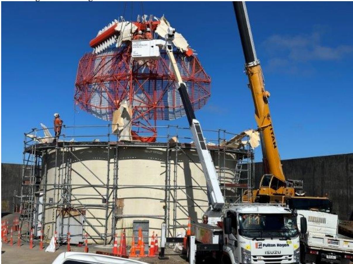
Removing THALES PSR/MSSR antenna
