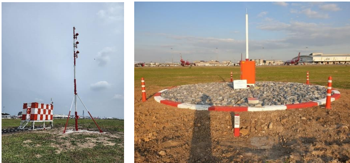
Figure 4. GBAS shelter and VDB antenna (left) and RR antenna (right) installed at Suvarnabhumi International Airport
