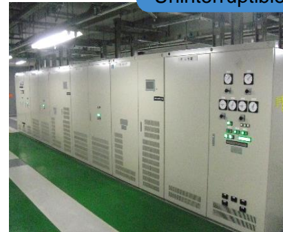
Uninterruptible power supply equipment
