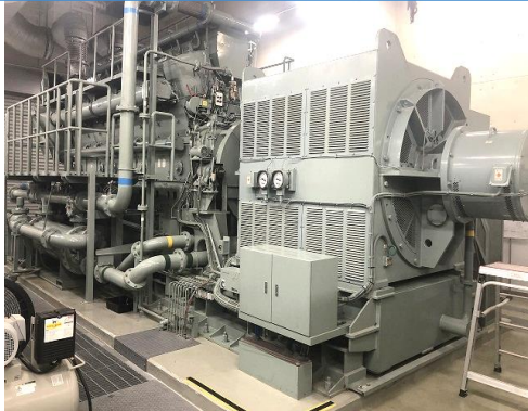
Emergency power generation equipment
