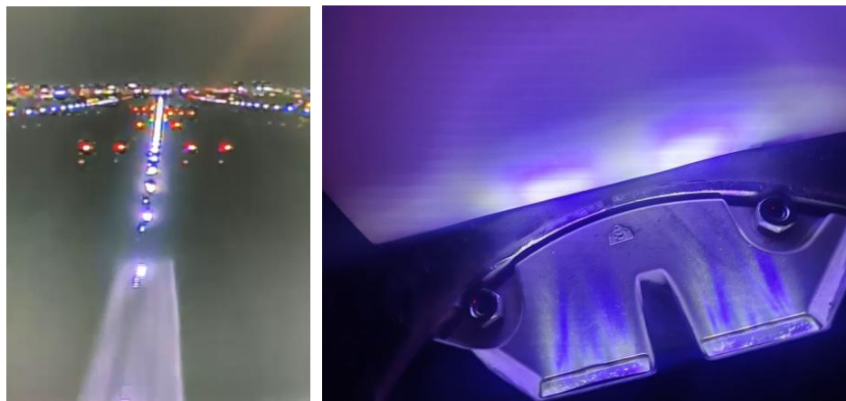
Fig 2. Typical color shift symptoms observed in runway centreline lighting (source: Anonymous)
