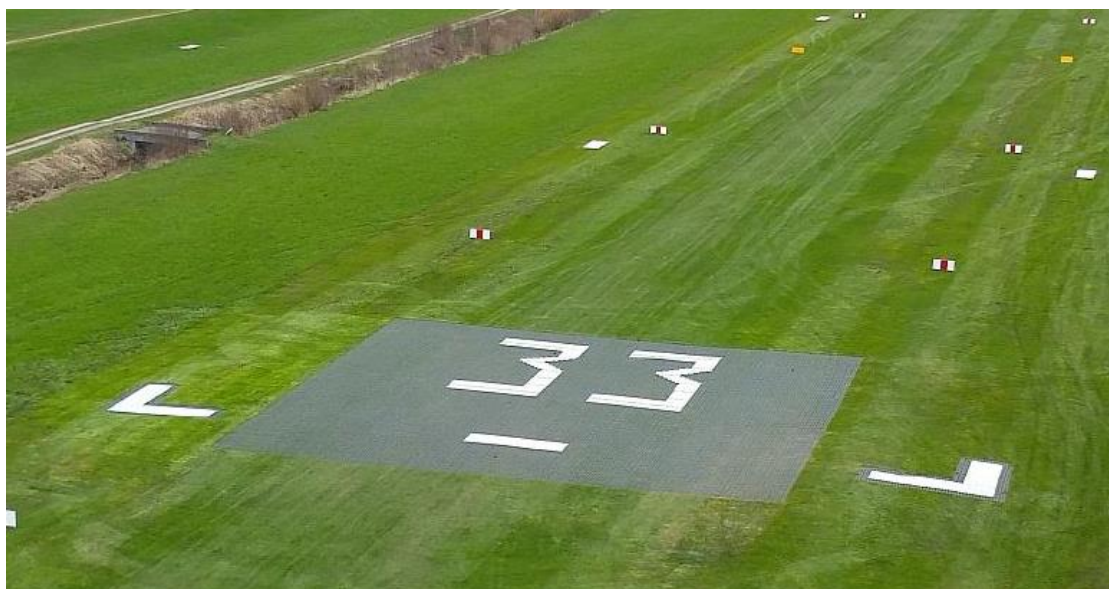
Figure 5 – 3: Example of Runway and Threshold markers
