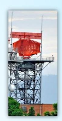
SSR coverage standard 250 NM but limited due terrain shadowing
