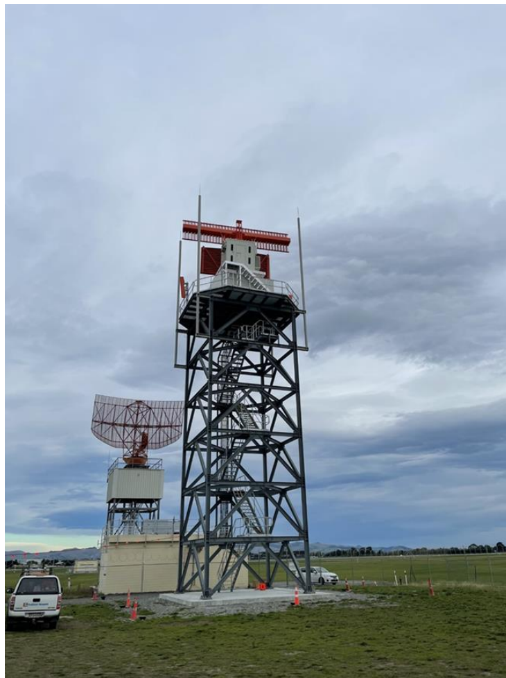
New INDRA MSSR/PSSR in front of old Thales PSR
