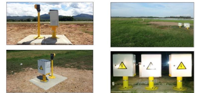
Mounting Support with SFL Power Equipment Cabinet Installed at Thailand Airports
