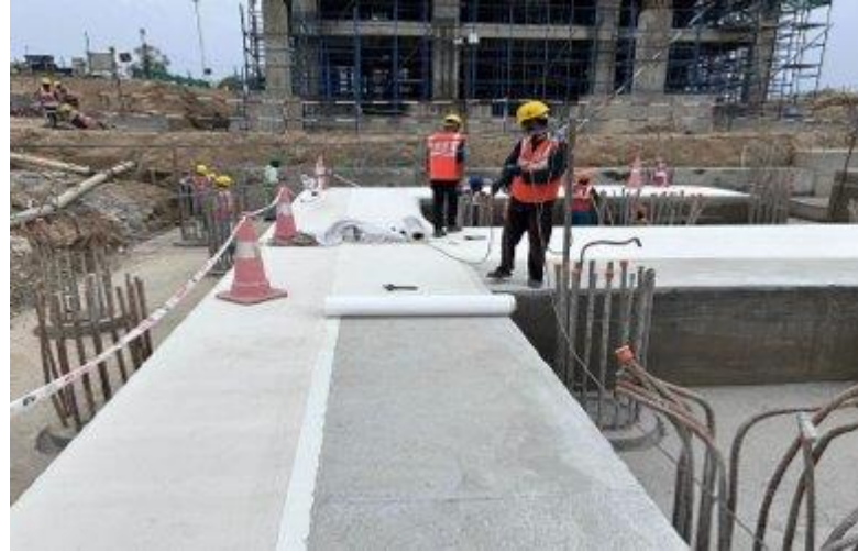
ARFF CLSM/PCC and Waterproofing Works
