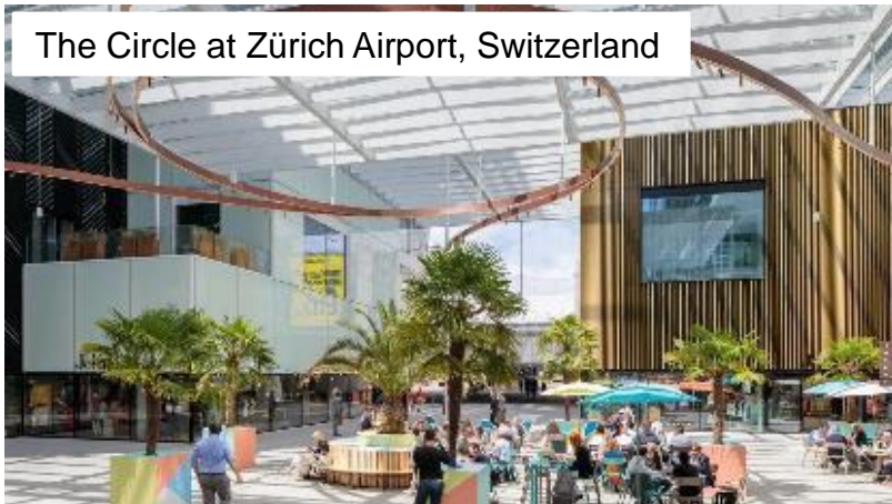
A complex incorporating retail, hotel and convention center, and office functions
