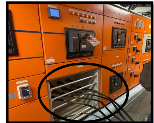
Quick hook-up to large-capacity mobile genset
