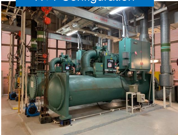
Water-cooled Chiller System (WCC)
