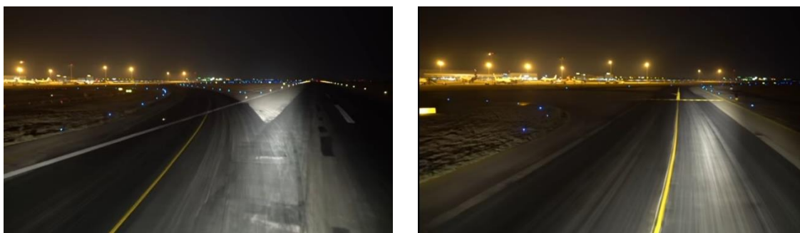
Figure 3. Aircraft identifying the Taxiway centre line marking from runway exit through its lighting
