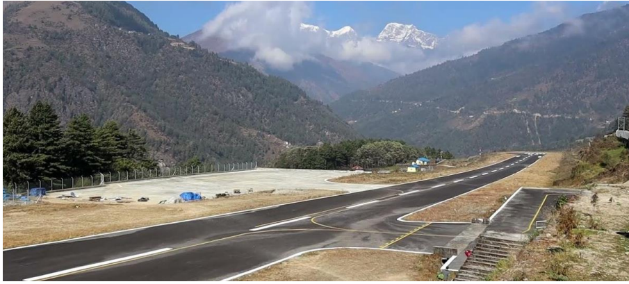
Figure 5 – 1: Runway marking at Phaplu Airport, Nepal
