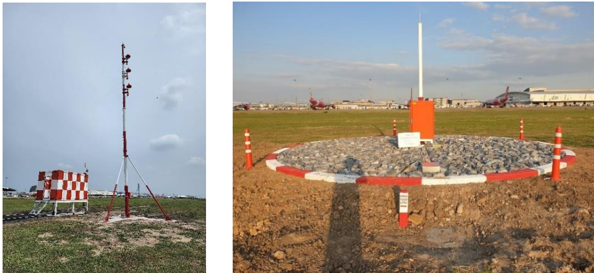
Figure 3. GBAS Shelter and VDB antenna (left) and RR antenna (right) installed at Suvarnabhumi International Airport
