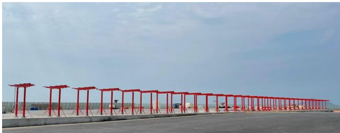
32-element wide-aperture localizer antenna array
