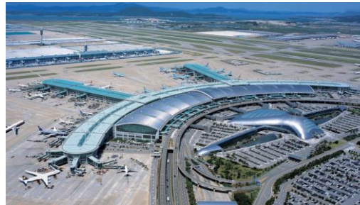
Total Airport Management System
