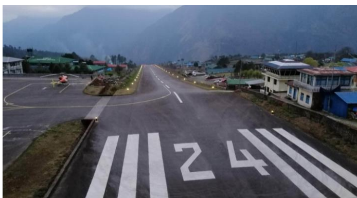
Figure 5 – 2: Runway Lighting at Tenzing Hillary Airport
