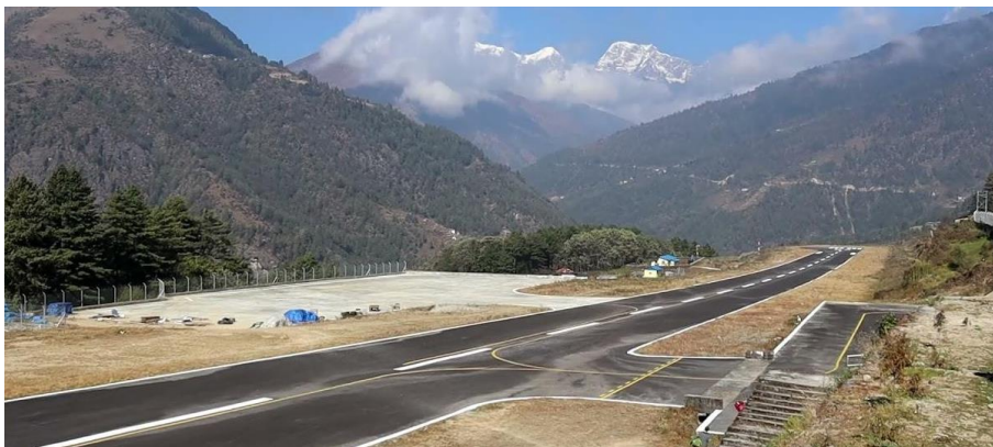
Figure 5 – 1: Runway marking at Phaplu Airport
