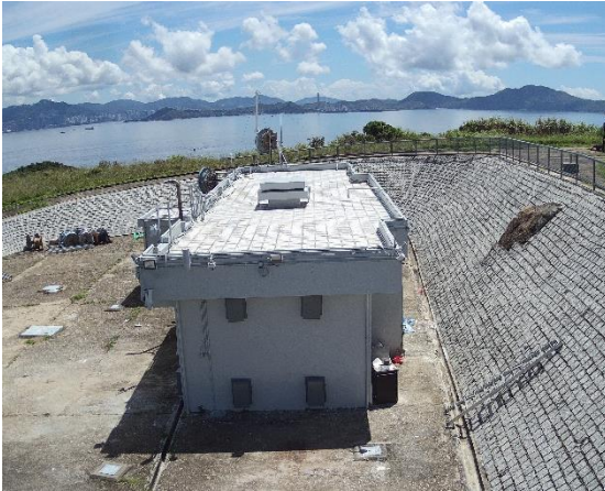
Figure 7. Image of Site Building by Drone
