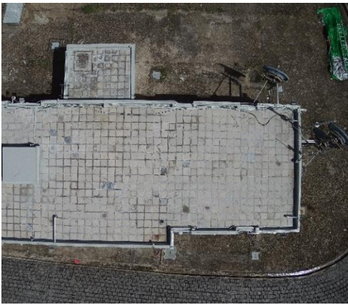
Figure 9. Image of Building Roof-top by Drone
