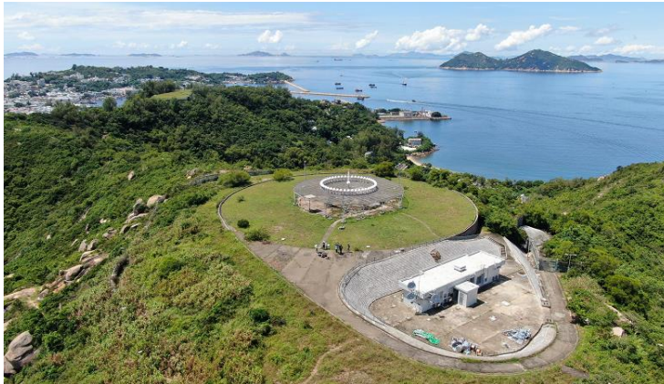
Figure 1. Overview Photograph of Cheung Chau Outstation taken by Drone
