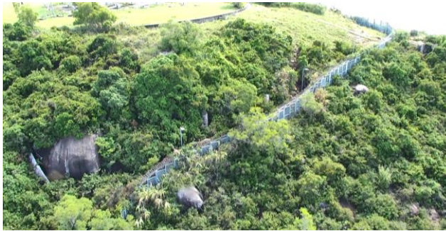
Figure 3. Use of Drone to Inspect Security Fencing along Steep Slope
