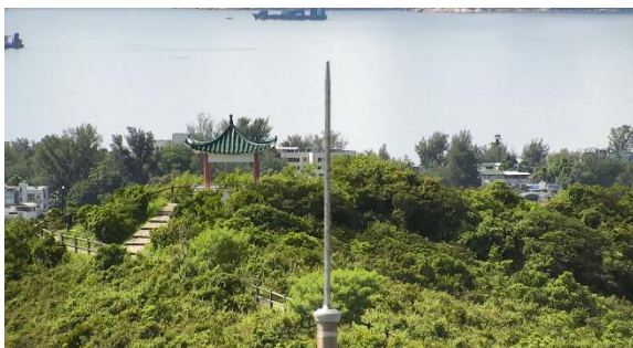
Figure 5. Close-up Inspection of Lightning Rod by Drone
