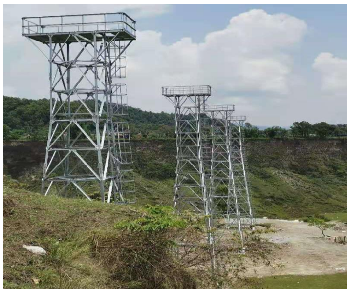
Figure: 3 Towers for installation of approach light barrettes
