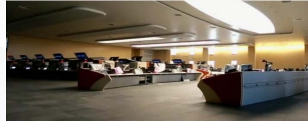
Air Traffic Control System with 170 Seats (biggest in China)
