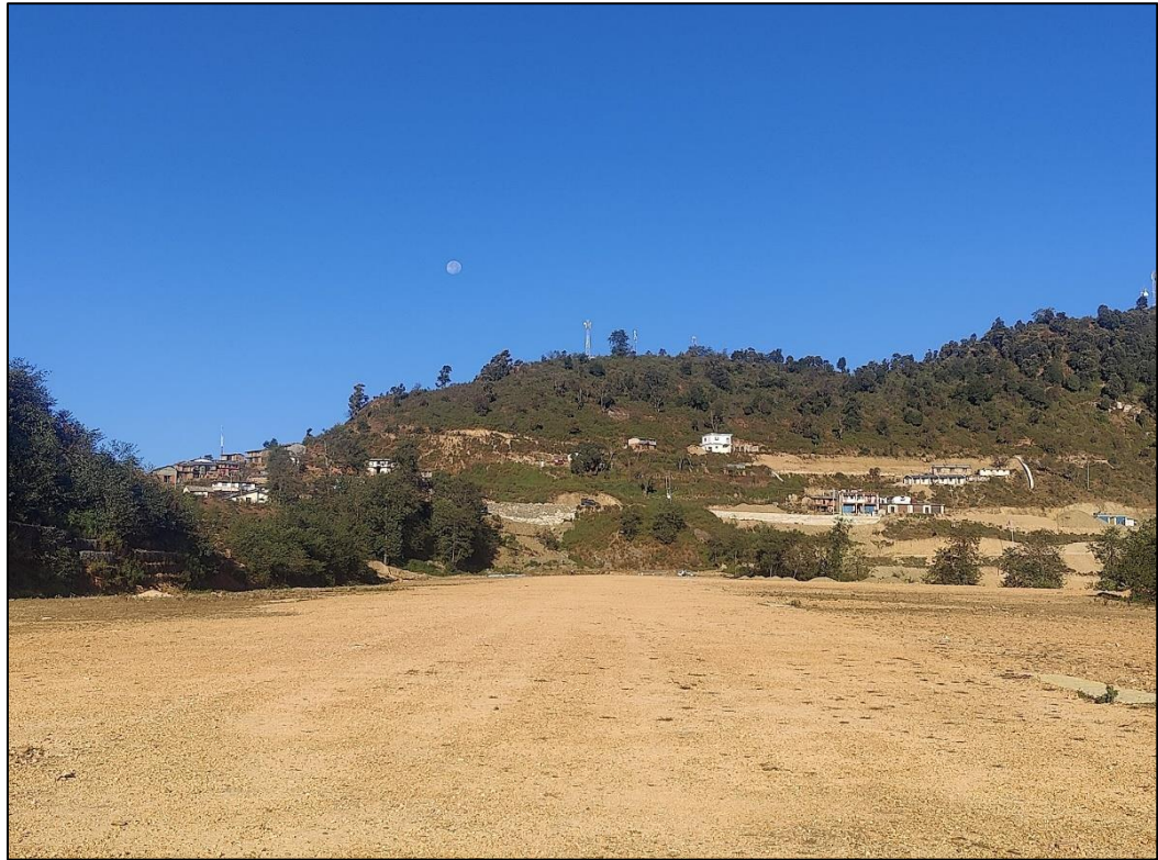
Figure 6.1 – Unpaved runway well graded and compacted
