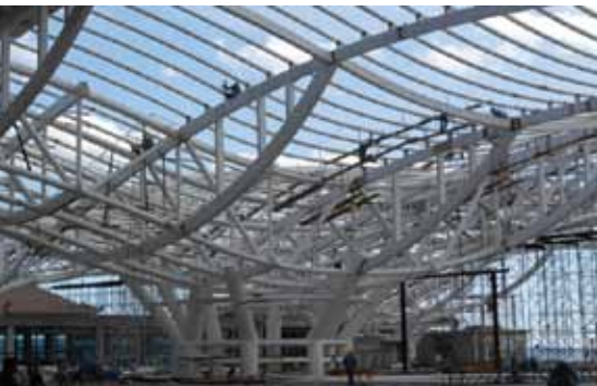
New terminal building at Denpasar Airport, Bali, currently under construction
