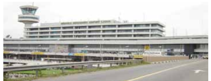
The main terminal building at the Murtala Muhammed International Airport in Lagos.
