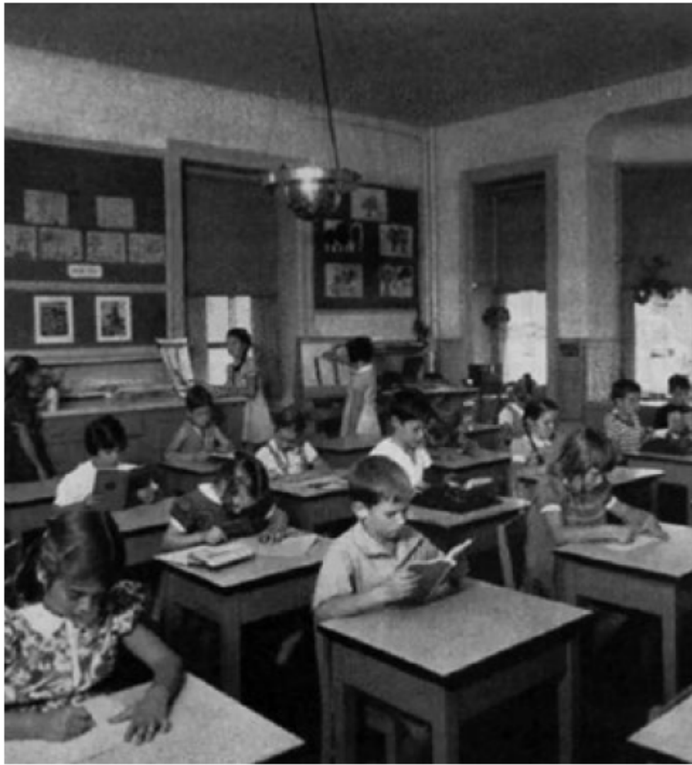
FIGURE 1.5. Picture from the Wells' study using GUV in the upper room portion of school classrooms 35 . The metallic chandelier holds UV lamps. These lamps point upwards, irradiating the unoccupied upper section of the room, relying on air circulation to move pathogens up and clean air down.
