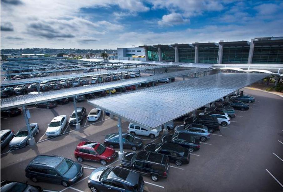
Results (Environmental Benefit/Cost Benefit): With the new solar photovoltaic arrays, SAN is annually generating approximately 9.3 million kWh of renewable electricity on site (about 20% of the Airport's total energy consumption).
