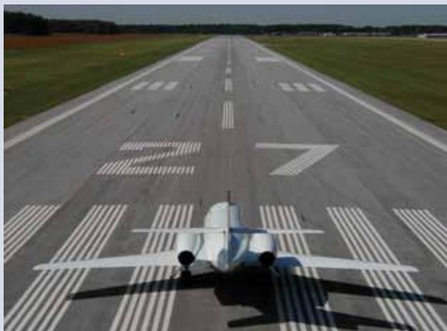
The Earth's magnetic field is constantly wavering and has finally shifted so far toward Russia that the magnetic alignment of airport runways in Florida, U.S.A., recently had to be re-numbered. The Tampa runways were closed early in 2011 for this purpose and to update taxiway signs.
