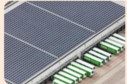
ASDA – UK (6.6 MW)
