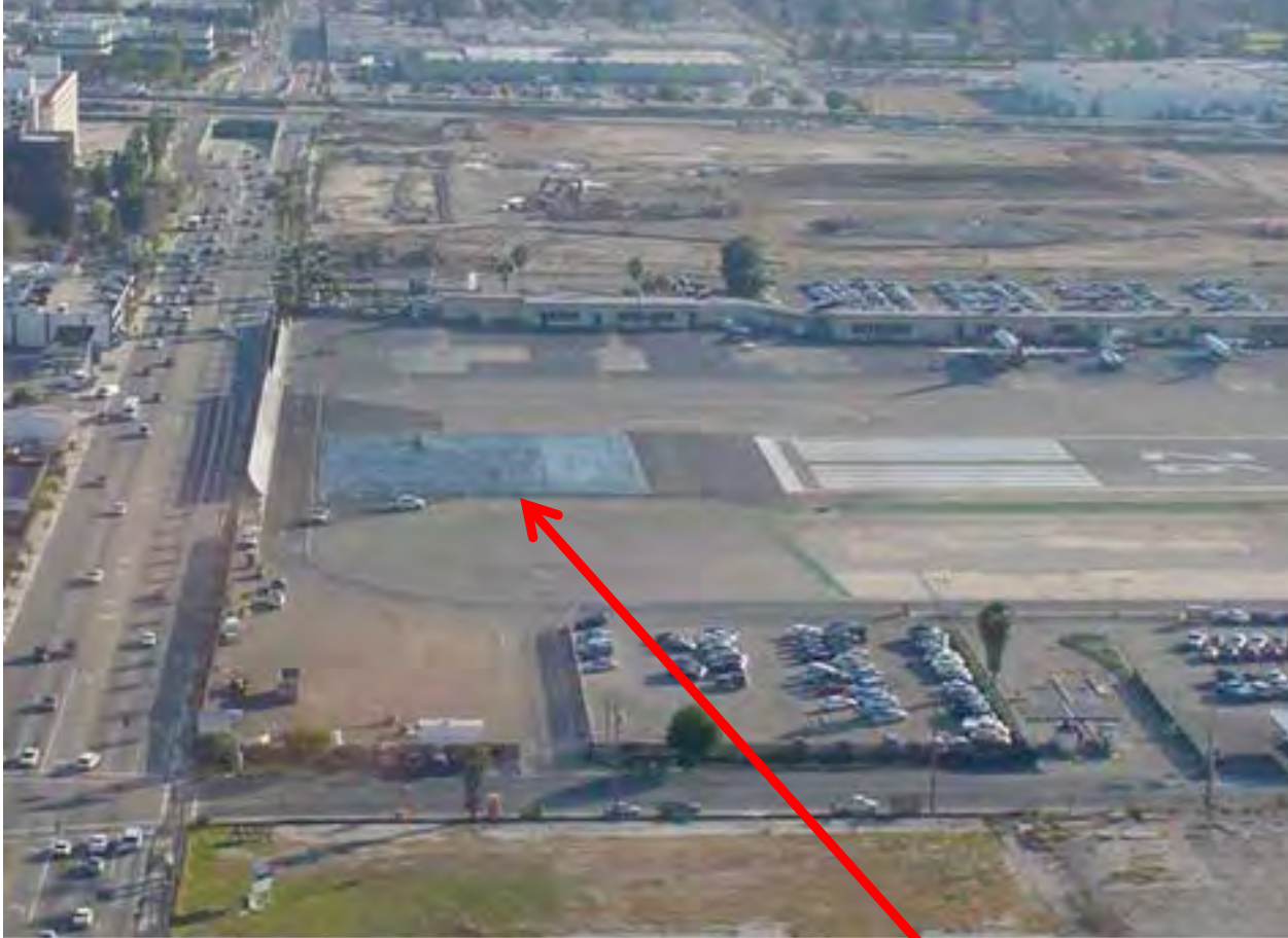
Aerial photo showing Hollywood Blvd. off Runway 26 at Burbank Airport, Burbank, California. EMAS installed for runway excursions
