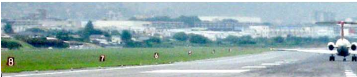
Figure 2. Distance remaining signs along a runway; close-up view of an individual installation
