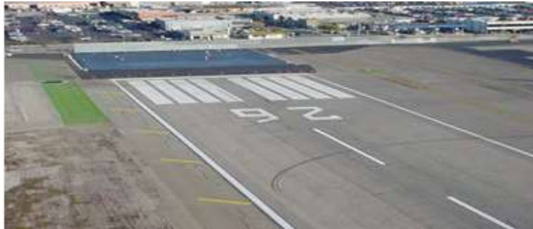
Figure 4. Aerial photo showing the original, materially-designed arrestor bed system installed off Runway 26 at Burbank Airport, Burbank, California
