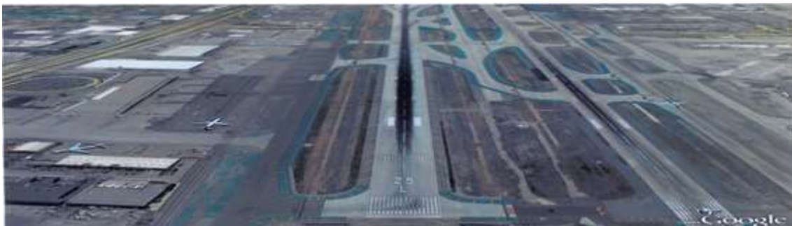
Figure 1: Excessive rubber buildup on the runway
