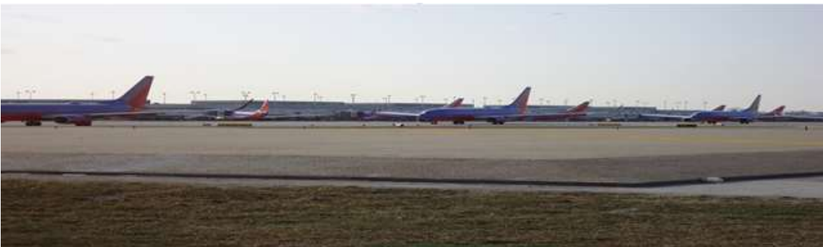
Figure 5. Ground photo showing the newest, materially-designed arrestor bed system installed off Runway 22L at Midway Airport, Chicago, Illinois
