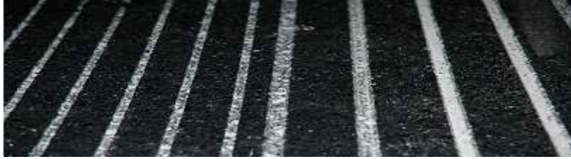
Figure 3. Standard (Left) and Trapezoidal (Right) Grooves Side by Side
