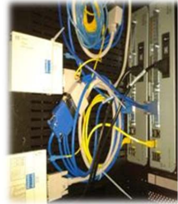
Optical fibre installation
