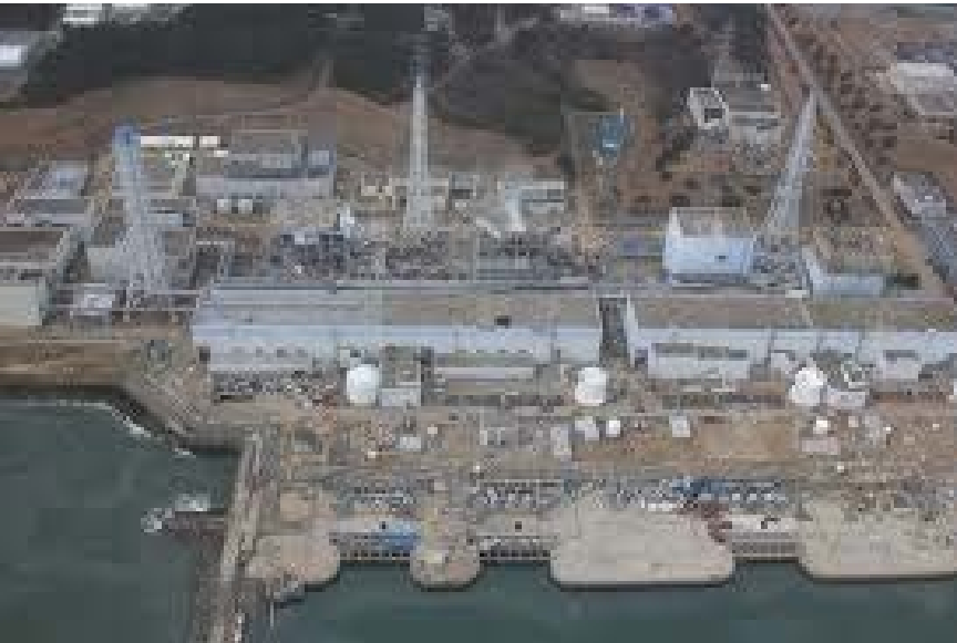
Fukushima nuclear facility (Mar 2011)
