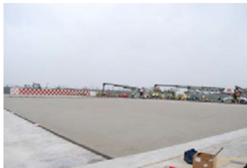
First EMAS installation by Runway Safe LLC, at Midway Airport.
