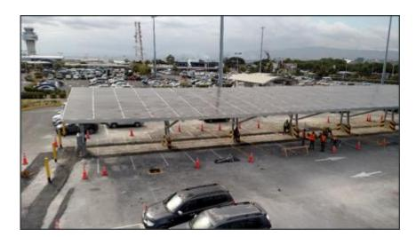
324 solar panels 100 kW Solar Photovoltaic System
