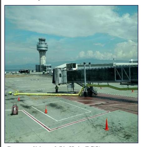
Pre-conditioned Air Unit (PCA) & 400 Hz Ground Power Unit (GPU)at Gate 1 Allows aircraft to plug-in to Terminal
