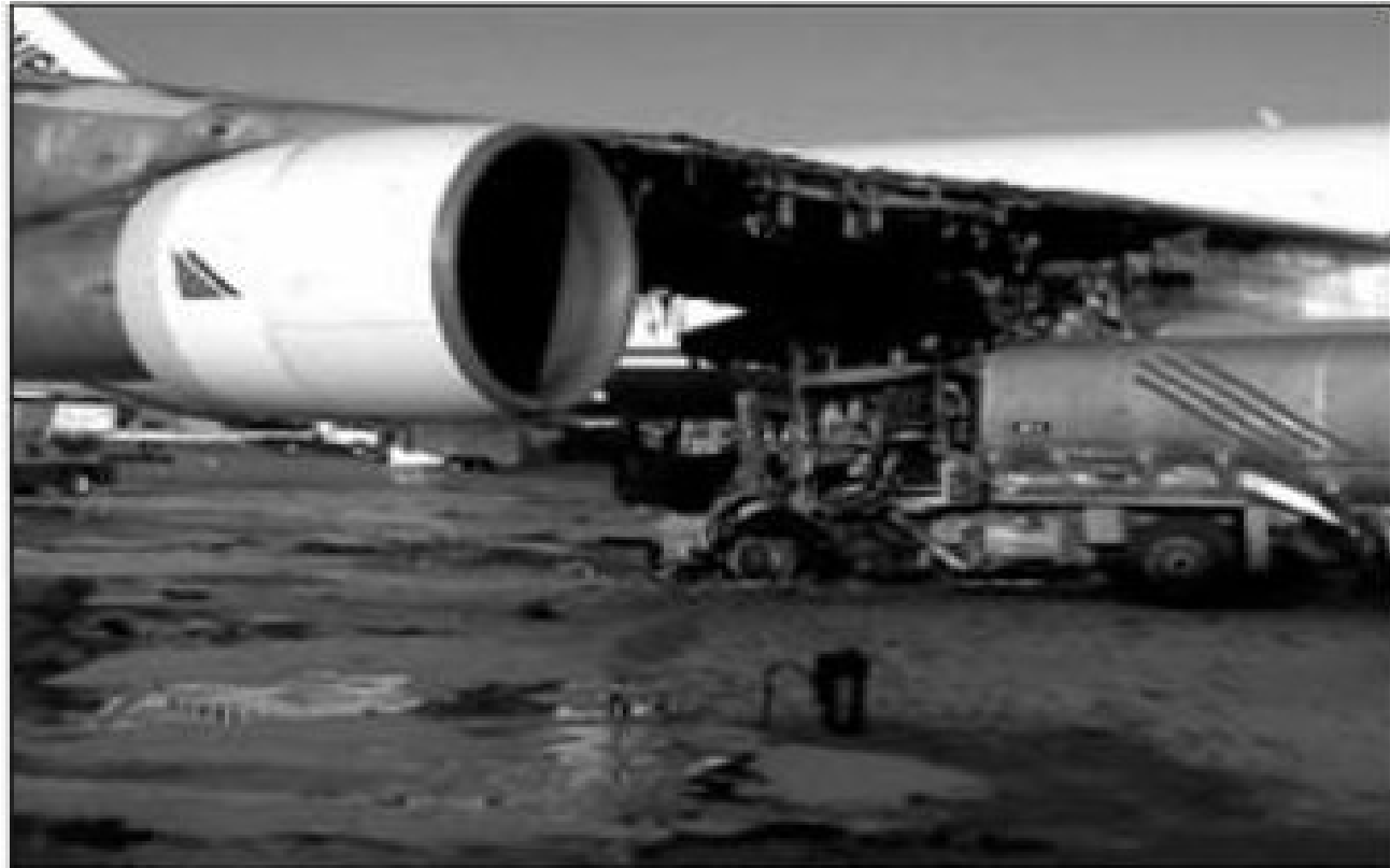
A Boeing 747-259B received substantial fire damage to the right wing during refueling Dec. 1, 1998, at Miami International Airport, Florida, U.S. (Photograph by Timothy Swick)
